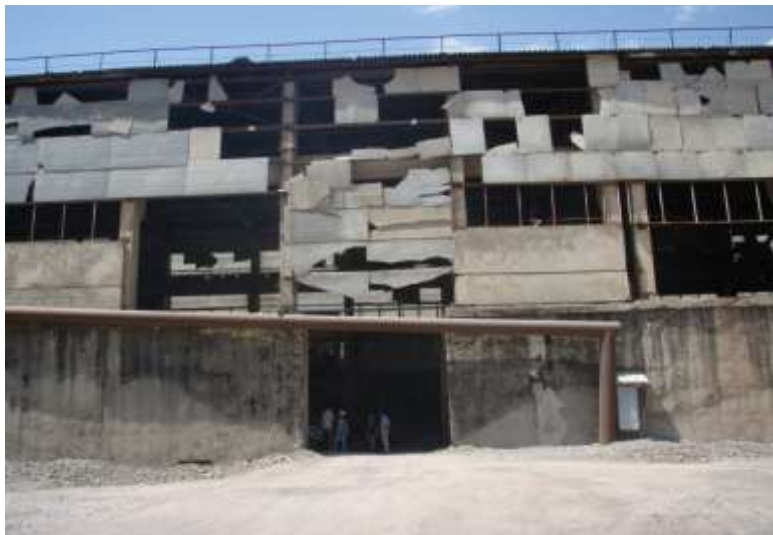
Figure 18-1: Breaker hall with largely damaged asbestos boards
