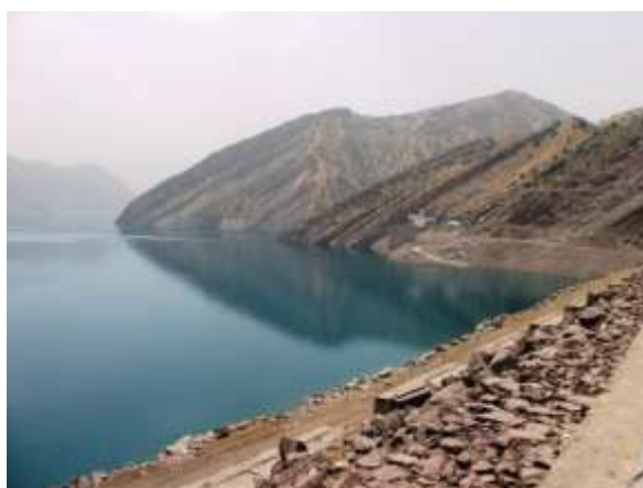
Figure 8-14: Nurek reservoir from dam crest
